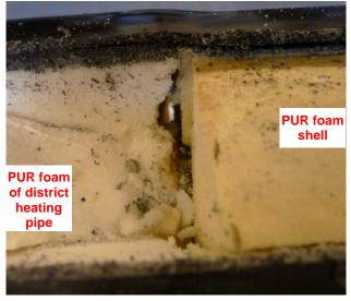
Figure 20. PUR foam is cut very irregularly, so that the PUR foam shell does not fit tightly, which leads to large gaps.
