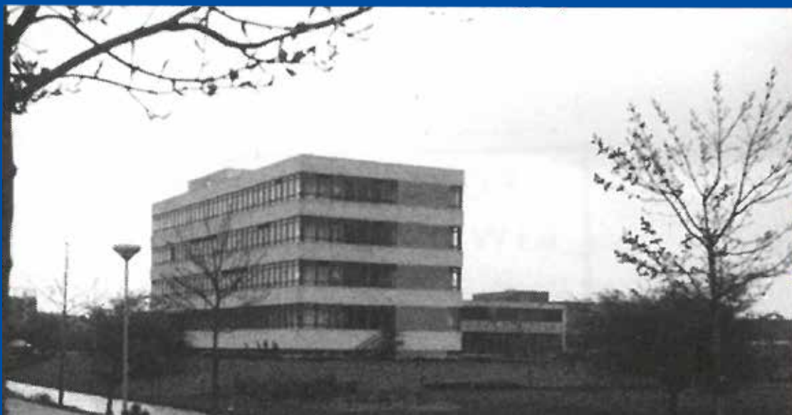
Kiwa building on Sir Winston Churchillaan, Rijswijk, the Netherlands 1965.
